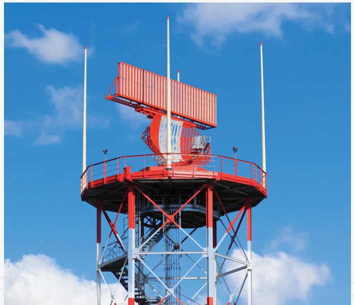
Co-mounted MSSR and passive ADS-B system
